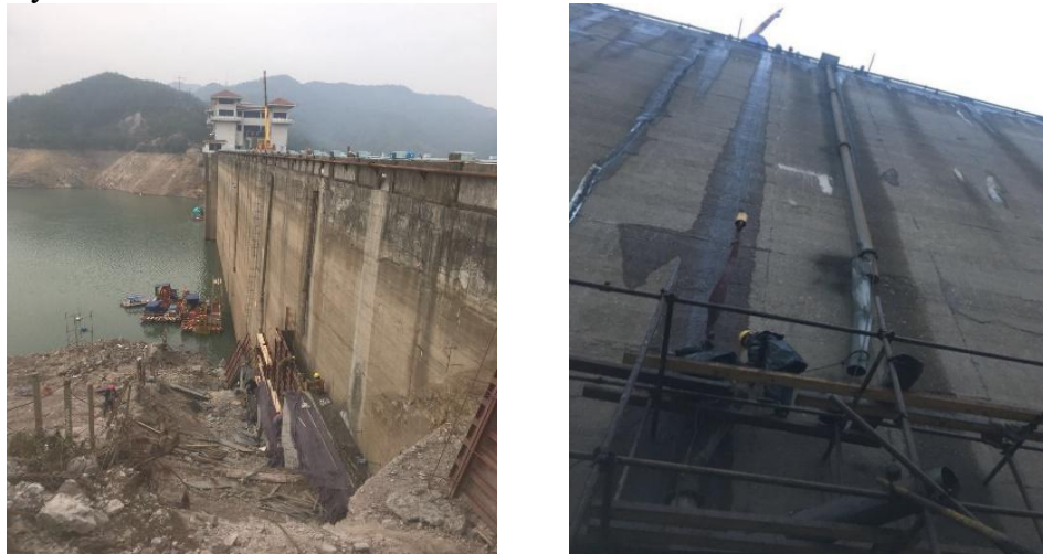
Figure 1: Construction of underwater concrete pouring in Wanyao Dam in Zhejiang.
